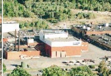
Sibbhult Gearbox manufacture and assembly.
